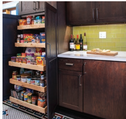
Rollout Trays in Tall Cabinet
